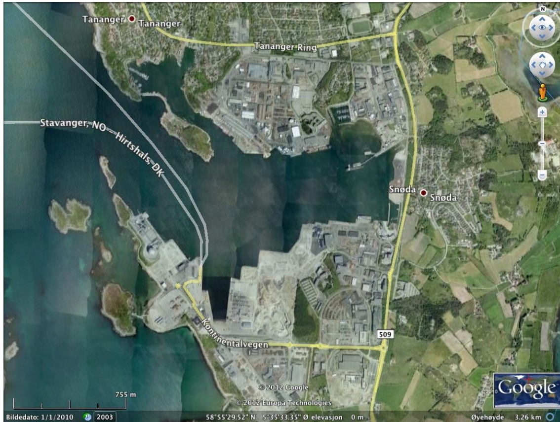
Figure 1: Satellite photo of the Risavika Area
