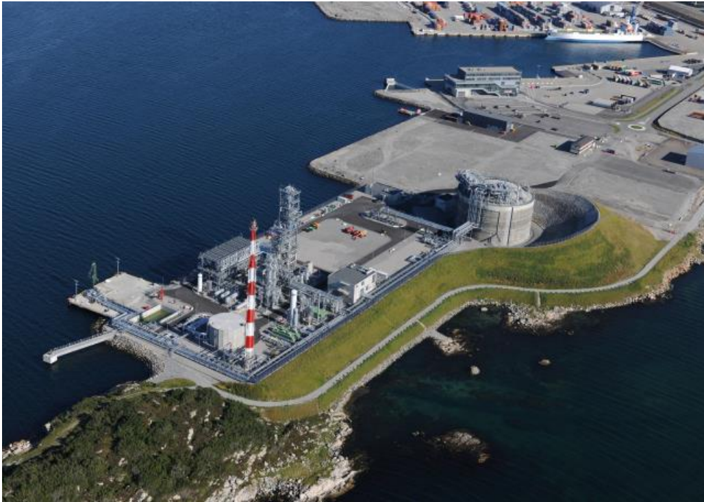
Figure 2: Skangass Plant at Risavika
