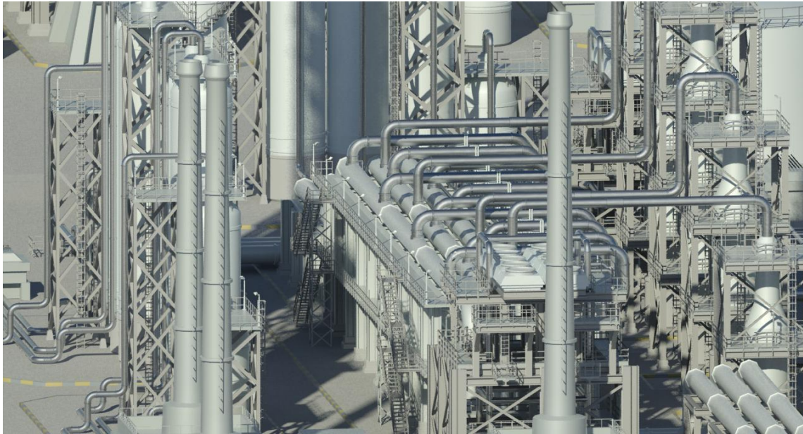
Figure 15 View of production site at CHEMCO facility.
