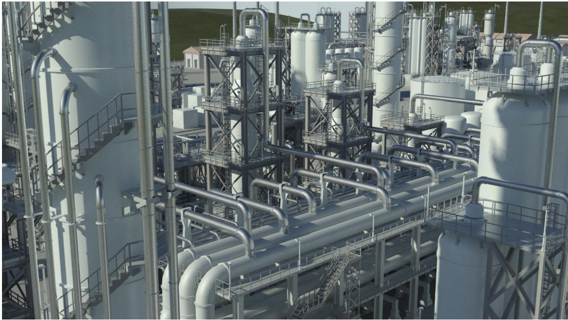
Figure 13 View of production site at CHEMCO facility.
