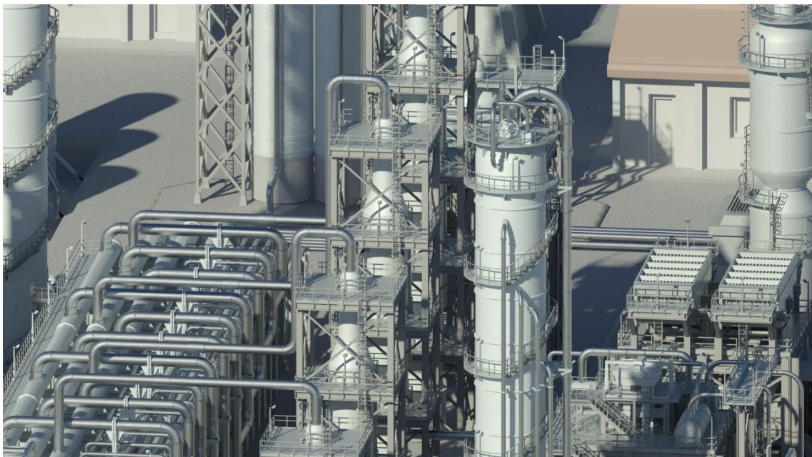
Figure 16 View of production site at CHEMCO facility.
