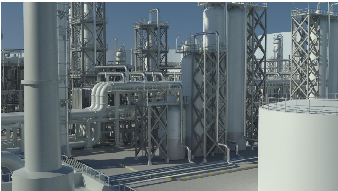
Figure 12 View of production site at CHEMCO facility.
