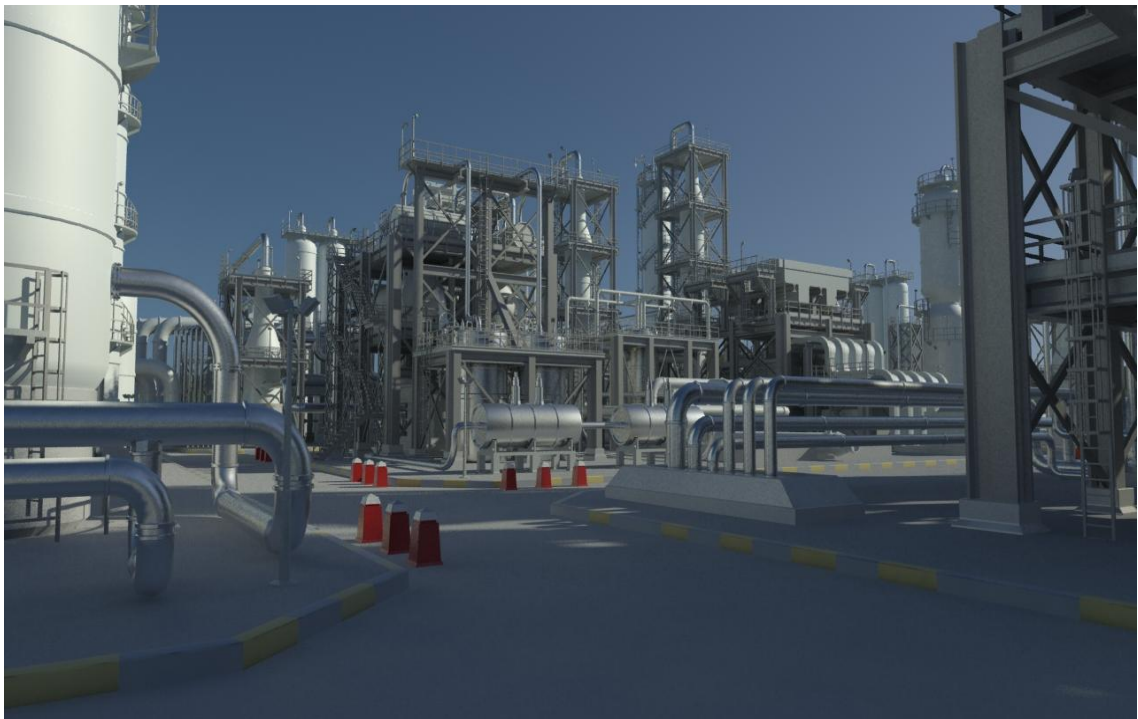
Figure 8 View of production site at CHEMCO facility.
