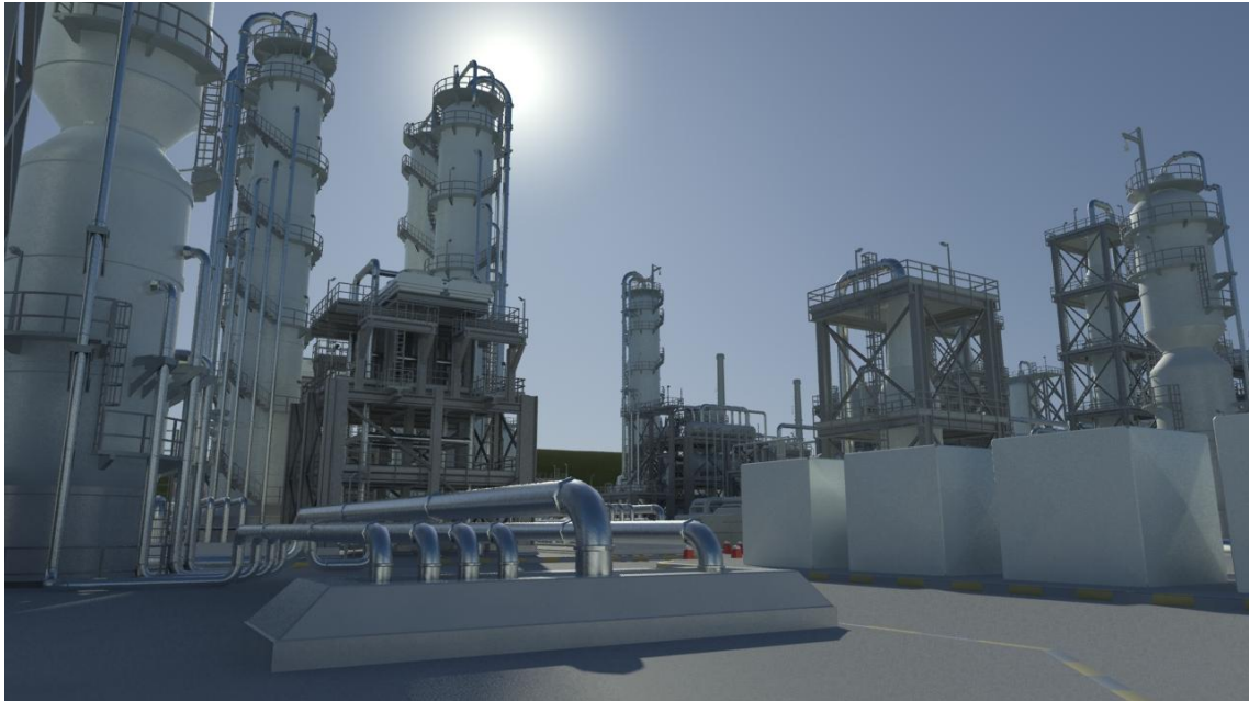
Figure 9 View of production site at CHEMCO facility.
