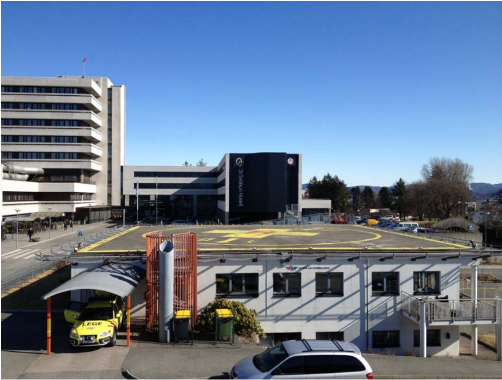
Part of the hospital
